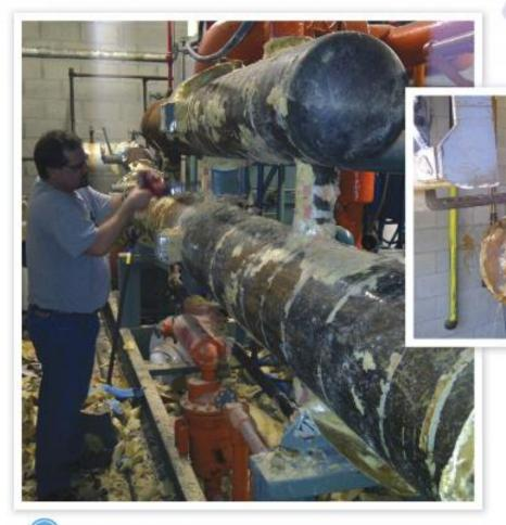
+ With the insulation off and the connections to the refrigeration system removed, it is time to take out the old chiller from the ice plant. The chiller is supported by chains in preparation for transport.
