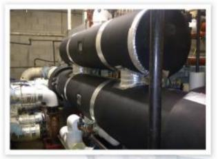
The final touch on the new chiller installation is insulating the package, and refilling with secondary refrigerant.
