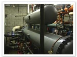
With all connections complete, the system is pressuretested, then charged with new refrigerant.
