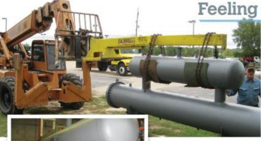
Bringing in the new chiller requires a boom fork with a heavy duty pencil extension. Fortunately for this crew, the ice plant has an overhead door, making the installation easier than most.
